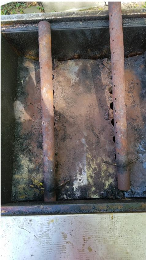
4. Remove the burner once clear of hole in the front wall.
